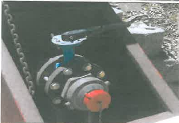
Water supply: Front standpipe, can be gravity fed from tank or pressurized by a pump
